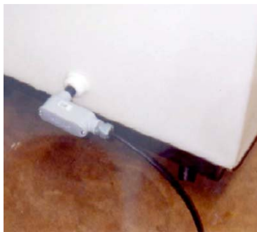
FIG. 6 Heater Conduit Boc Installed on Tank
